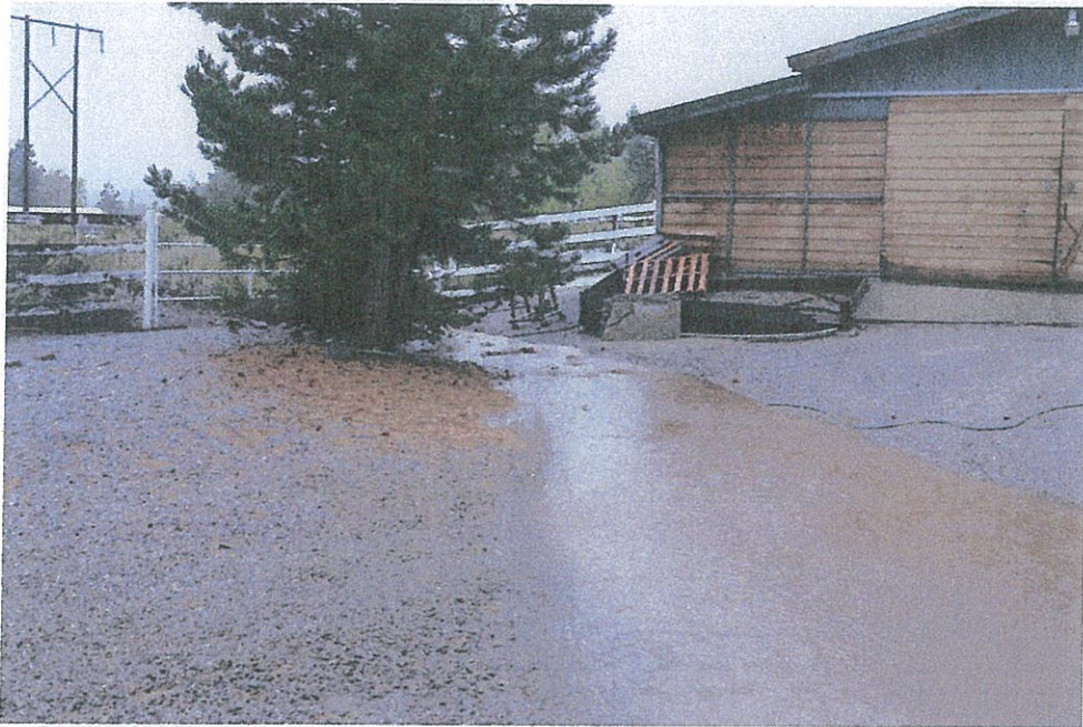
P3. Storm water from the proposed Sierra Village moving through private property.
