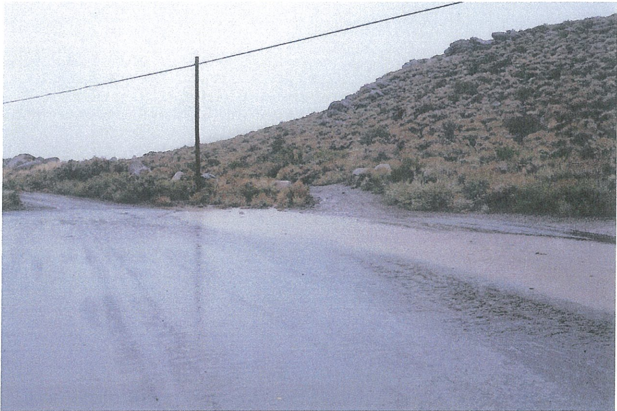
Storm water runoff from area of Sierra Village onto Cedarwood Drive October 16, 2016 5:39 PM.
