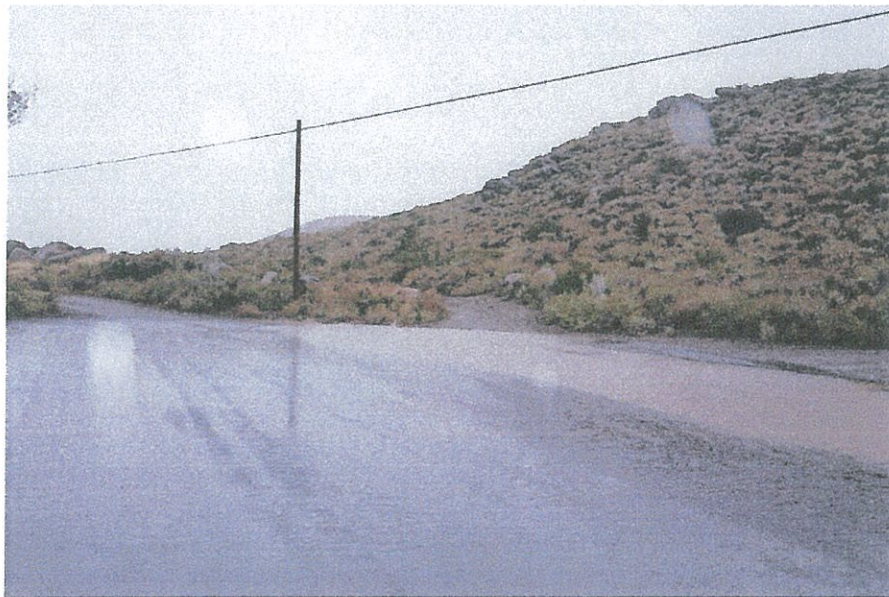
P2. Storm water draining onto Cedarwood Dr.
