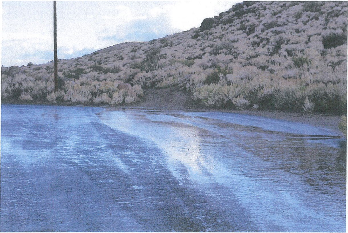
Storm water runoff from area of Sierra Village onto Cedarwood Drive October 16, 2016 8:27 AM.
